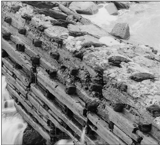
Detail of cribwork, showing concrete fill exposed along the top.
