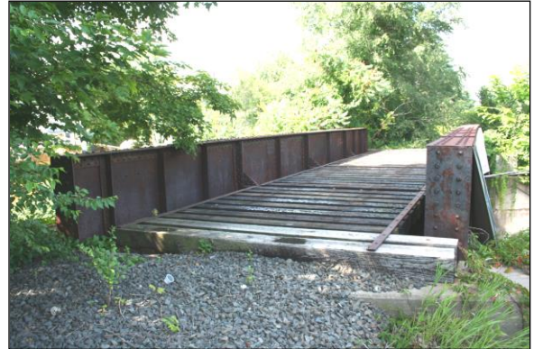
Plate-girder bridge, 1914, fabricated by Boston Bridge Works.
