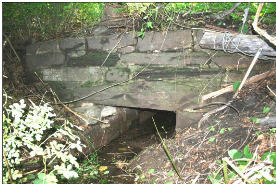
Brownstone box culvert, probably part of the original (1847) construction.
