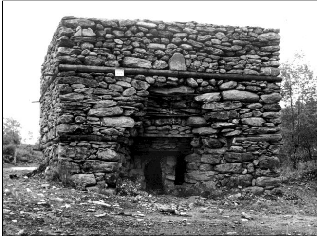
Mount Riga blast furnace structure
