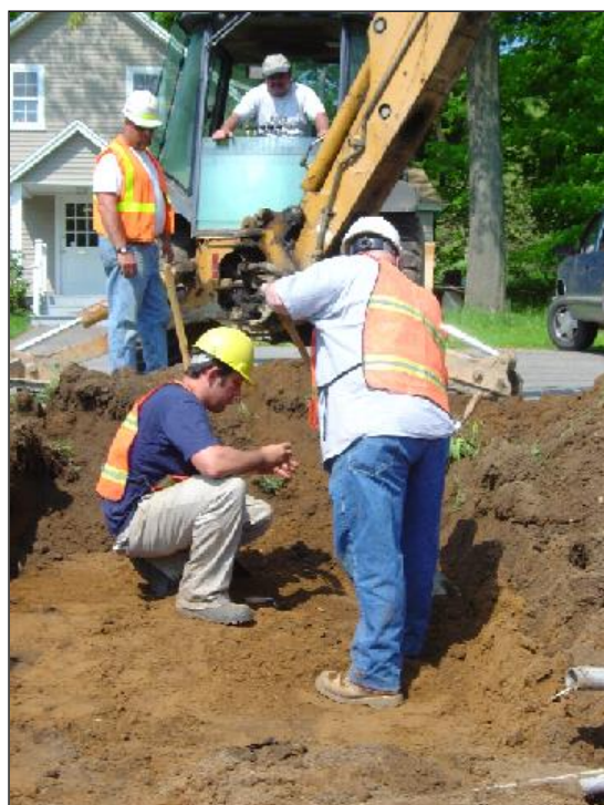
Topsoil Removal at Site 96-134
