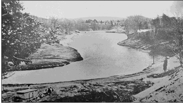
Main reservoir shortly after its completion in 1906.
