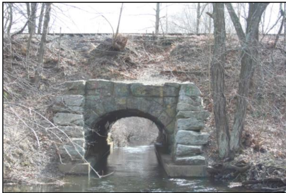
Assabet River railroad bridge, ca. 1852.
