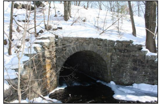
Cold Harbor Brook railroad bridge, ca. 1866.
