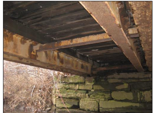
Former I-beam railroad bridge.
