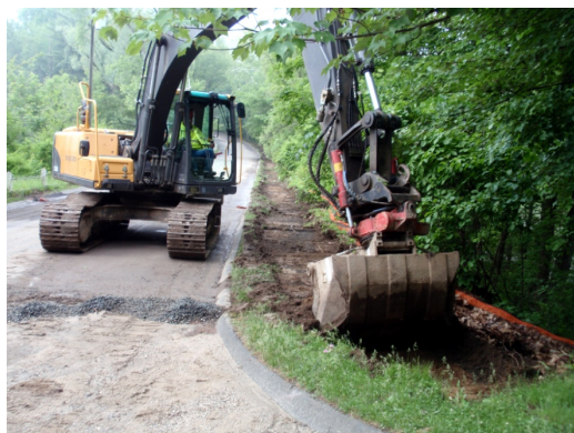
Archaeological monitoring of utility trenches
