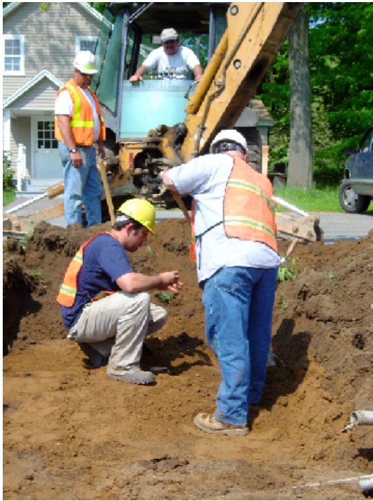
Topsoil Removal at Site 96-134
