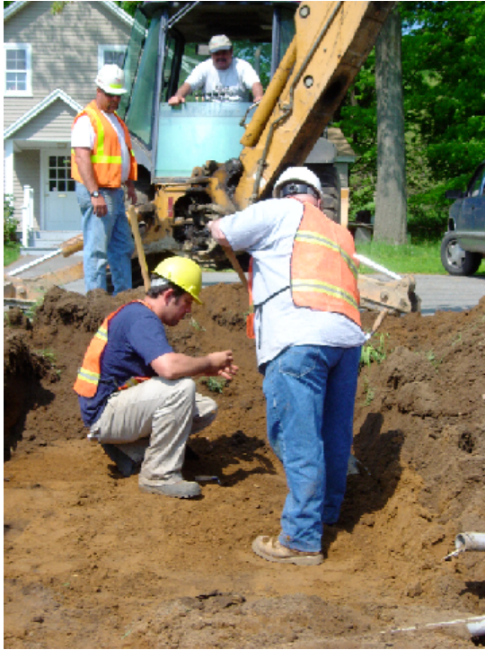
Topsoil Removal at Site 96-134
