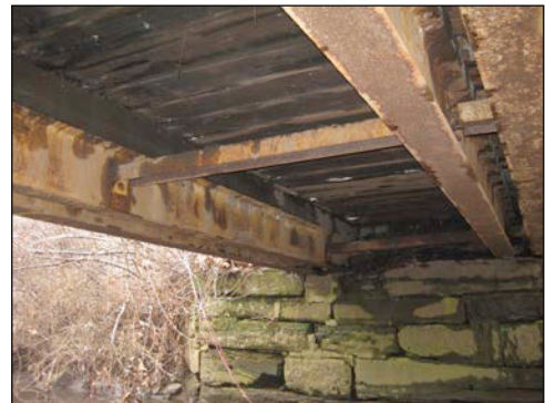
Former I-beam railroad bridge.
