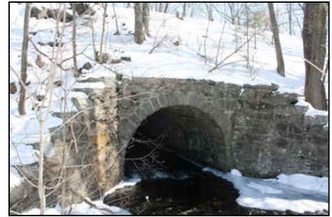
Cold Harbor Brook railroad bridge, ca. 1866.
