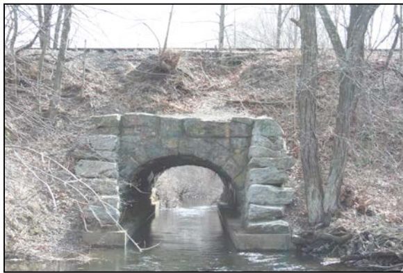
Assabet River railroad bridge, ca. 1852.
