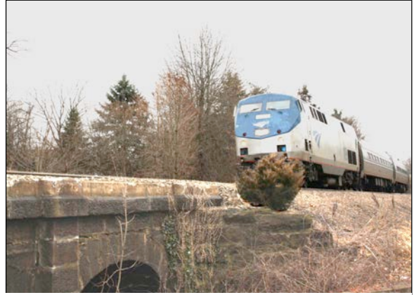
Many of the bridges along the corridor are stone arches, such as this 1870 example in Berlin, Connecticut.
