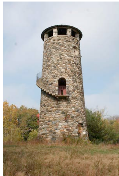
Stone Tower at Camp Columbia, built in 1942.
